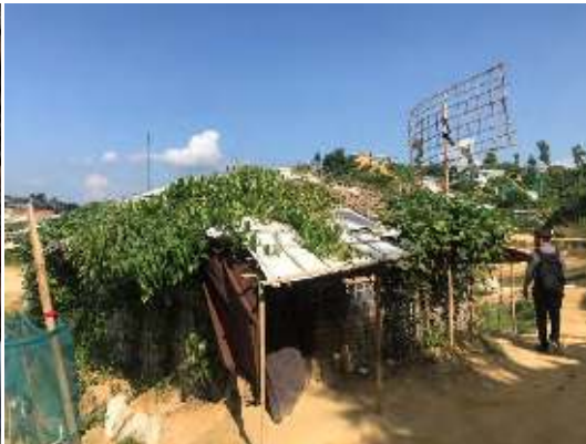
Example of green roofing
