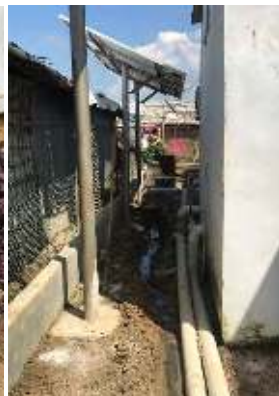
No proper drainage
