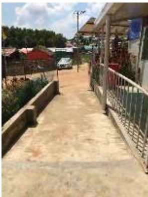
Camp 15 : Access ramp
