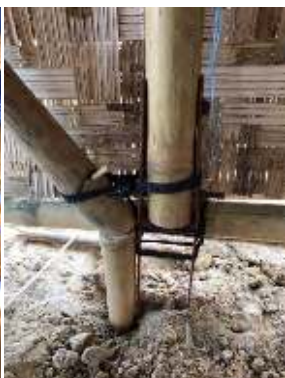
Detail of bamboo footing
