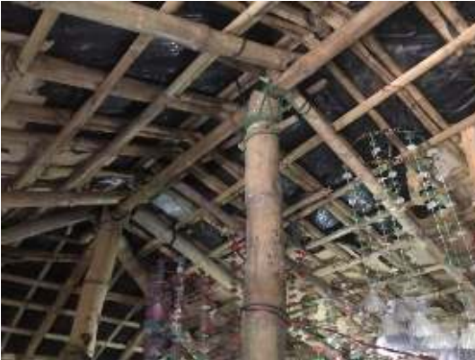
Bamboo connections
