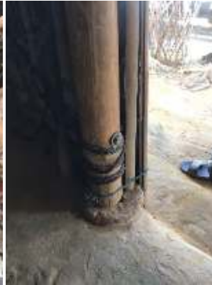
Medair's personal developed bamboo footing
