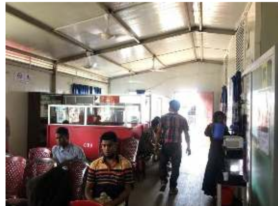
Interior (no visible bracings)
