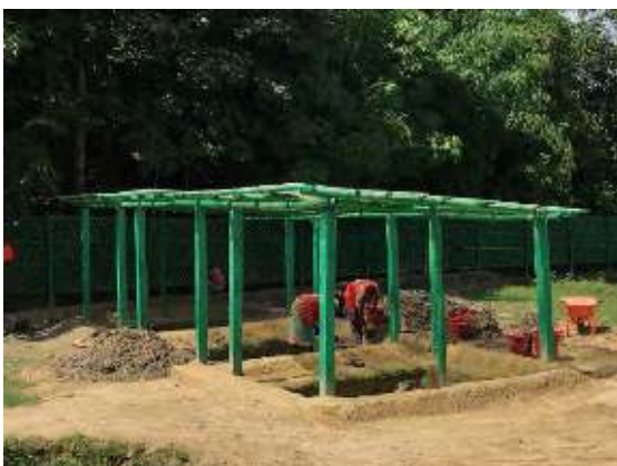
MRF Camp 15: Compost pits
