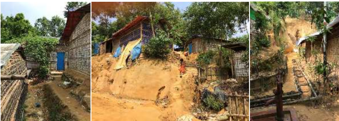
Camp 19: no drainage
