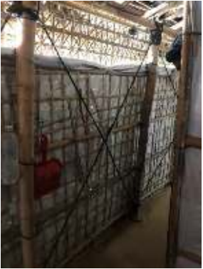
Upper wall ventilation and bracing details
