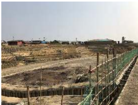
Site development: soil stabilisation & drainage
