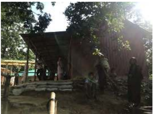
Slope stabilization needed (front side)
