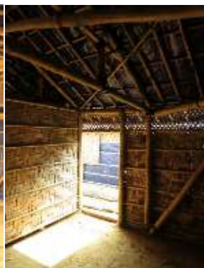
Door & lack of privacy
